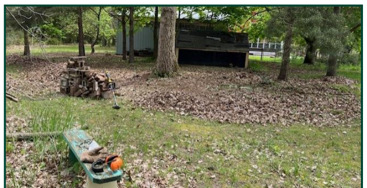
Gillan's second site under pine trees during rubble removal. Photo courtesy of Amy Gillan.
